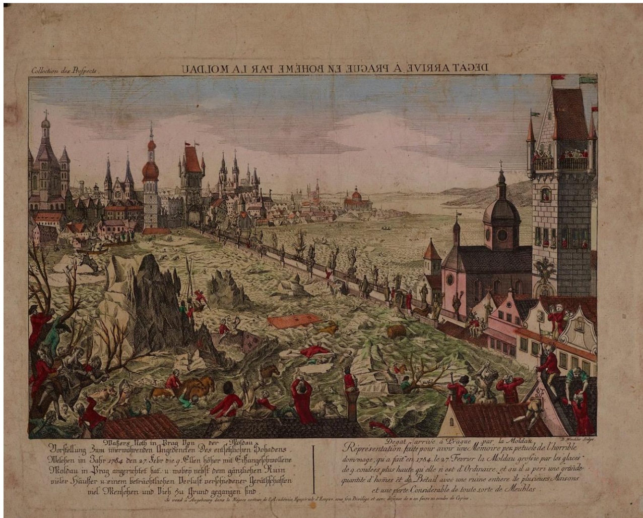
Fig. 1: The February 27, 1784 Flood of the Vltava River.
